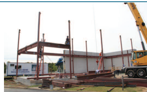
Structural steel work began Sept. 15.
